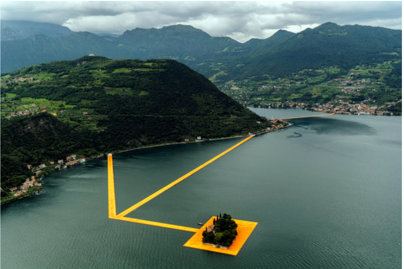
Figure 6.14 Project of artist Christo, The Floating Piers (2016) in Pilzone, Italy, that connects island on the lake by structure of 220,000 floating polyethylene cubes, covered of waterproof fabric. Photograph by Alessandro Grassani for The New York Times.
