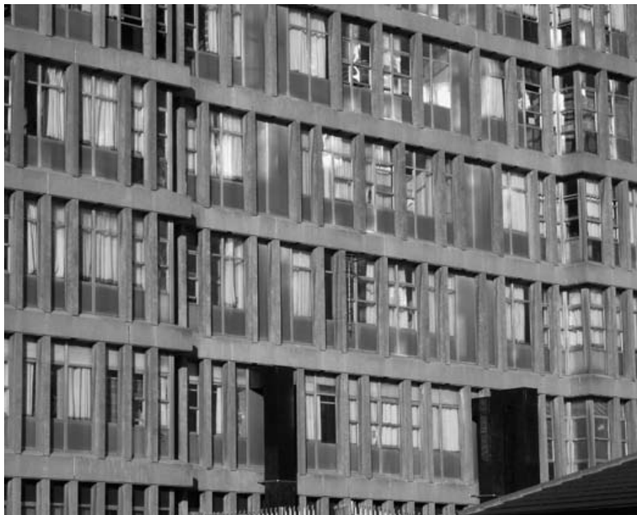
Figure 5. 5 Photograph of Northwick Park Hospital in London, 1961, by British architect John Weeks. Façade envelope was determined by computational algorithm having high and loading characteristics as a code. Photograph by David Theodore. Source: Architecture in Formation: On the Nature of Information in Digital Architecture (2010), p.74.
