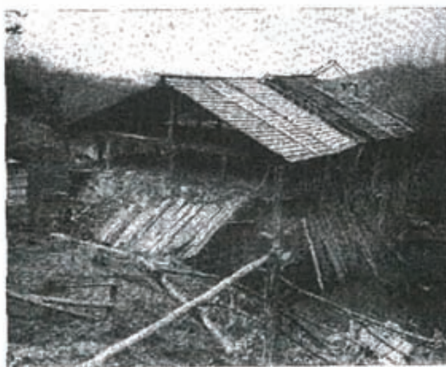
CENTRAL BARK DRIER WITH A CAPACITY OF SEVERAL TONS OF FRESH BARK THIS STRUCTURE WAS PLANNED AS A BUYING CENTER.
