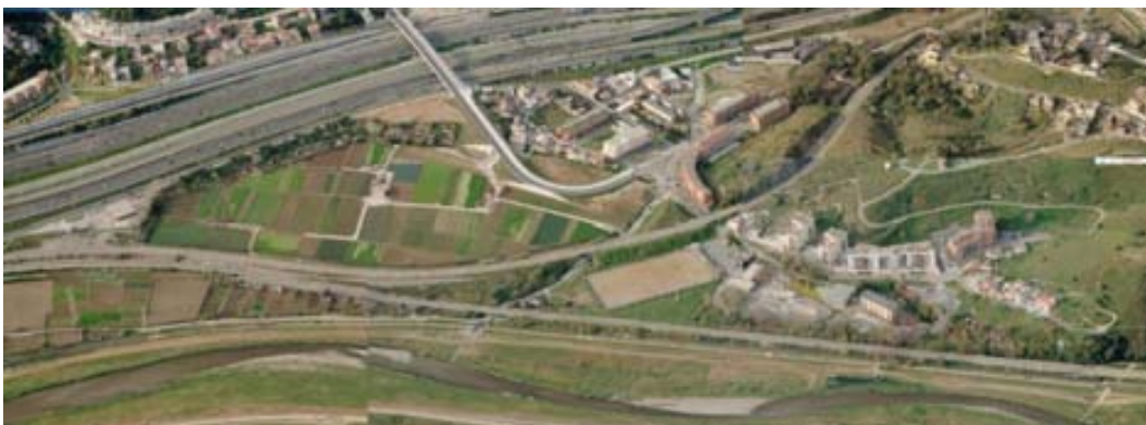
Figure 3.3. Aerial view of the neighbourhood location in Vallbona (Barcelona, Spain).
