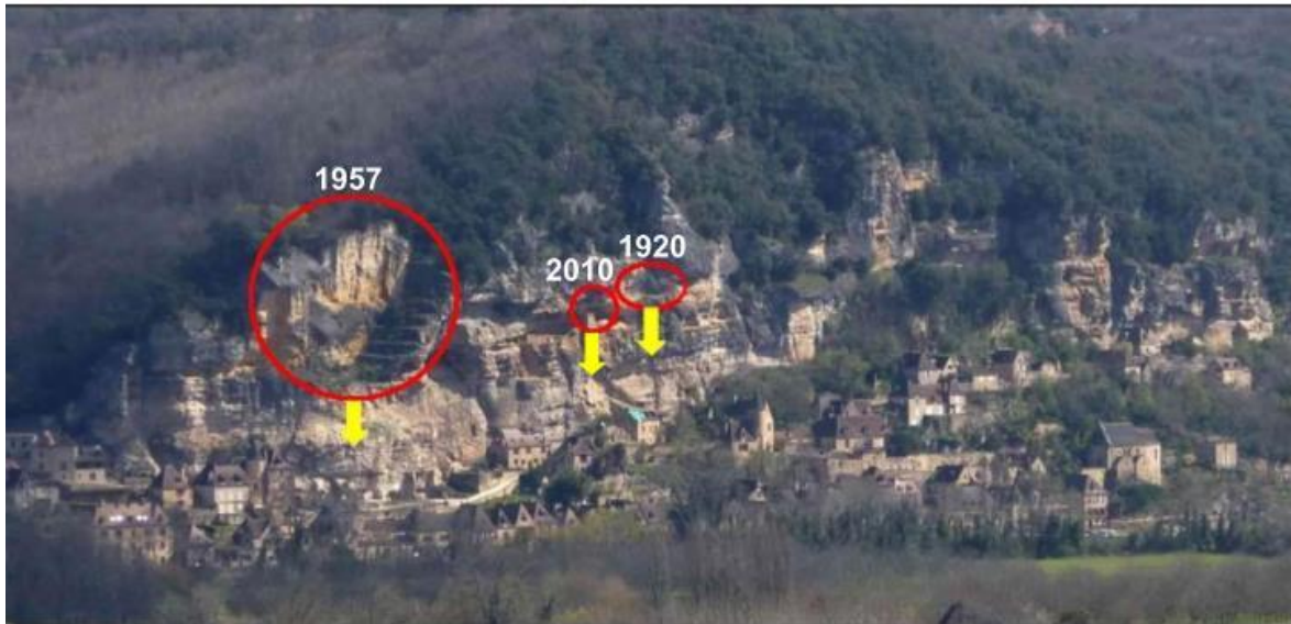
Figure 2-5 Location of principal events observed in the town (Virely and Guittard, 2010a)
