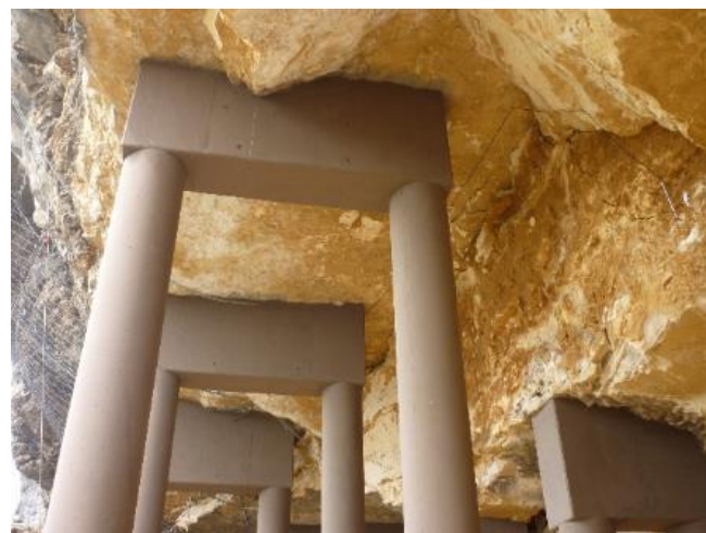
Figure 2-12 Supporting structures inside the cavern
