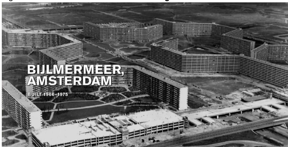
Figure 4.19: The construction of the buildings
