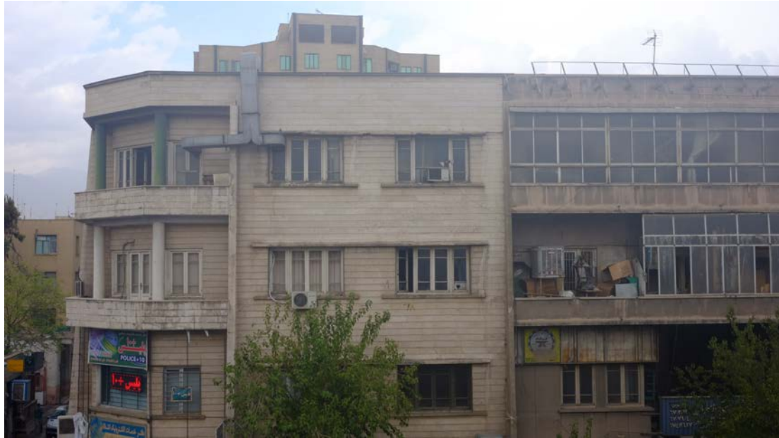
A common street-view in central Tehran, November 2015
