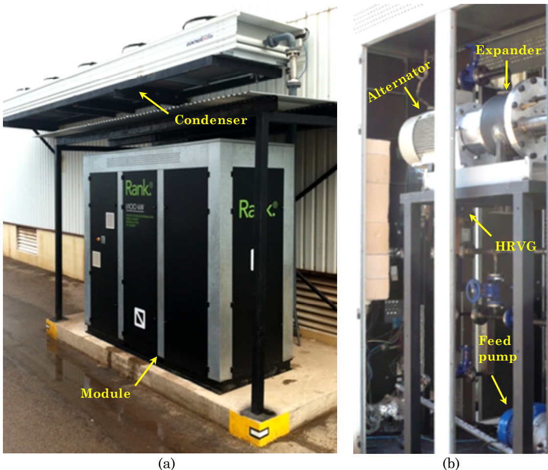
Fig. III.7. Photos of ORC: (a) external view of the unit (set of module and condenser), (b) internal view of the module.
