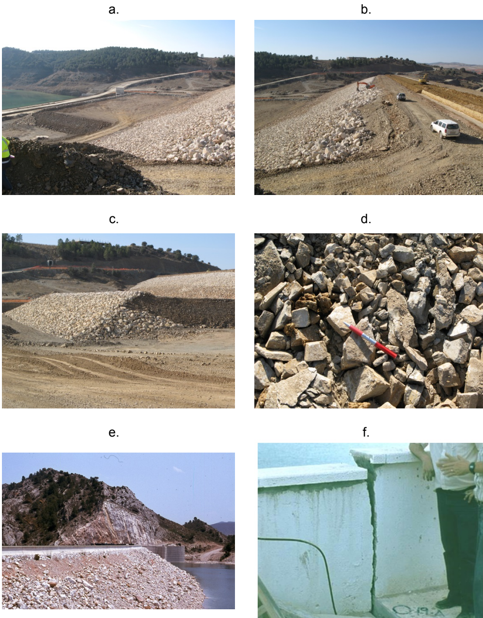
Figure 2-2 Rockfill dams: (a)-(d) Construction of Lechago Dam in 2008 (Spain): (a) Detail of rockfill in the shoulder upstream; (b) Detail of shoulder upstream and the crest of the dam; (c) Detail of rockfill; (d) Detail of slate rockfill. (e)-(f) Calanda dam in 1983 (Spain): (e) Detail of rockfill; (f) Detail of crack in the crest due to settlements (Photos are courtesy of the Professor E.E. Alonso).
