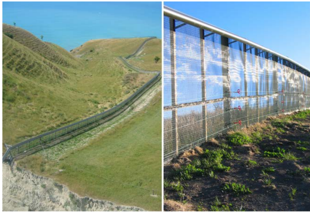
Image 2.40: The 1,640-foot-long Excluder Fence includes a flange at the top to discourage climbing rodents. A below-grade flange repels any attempt to dig under the barrier, Nelson Byrd Woltz, 2010.
