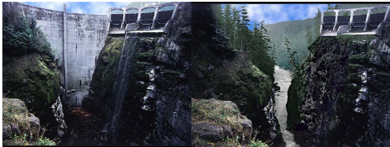
Image 2.28: The 210' concrete curtain of Glines Canyon Dam, Washington. Images of the dam's current state and rendering of post-dam removal, USA National Park Service, 2014.
