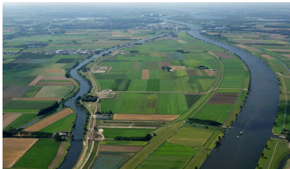
Image 2.46: Overdiepse Polder, an infrastructure project in the southeastern province of Brabant south of Amsterdam, will have eight elevated farms, CreditDick Sellenraad, 2013.
