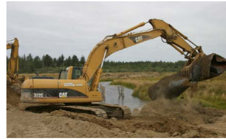
Image 2.55: A Knife River excavator crushes the Fahys Creek culvert shortly after it was extracted from the dike in the Bandon Marsh restoration , USFWS - Pacific Region, 2011.
