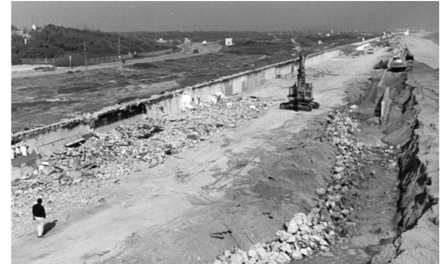
Image 1. 69: Construction on the promenade beach, LLORET, 1970.
