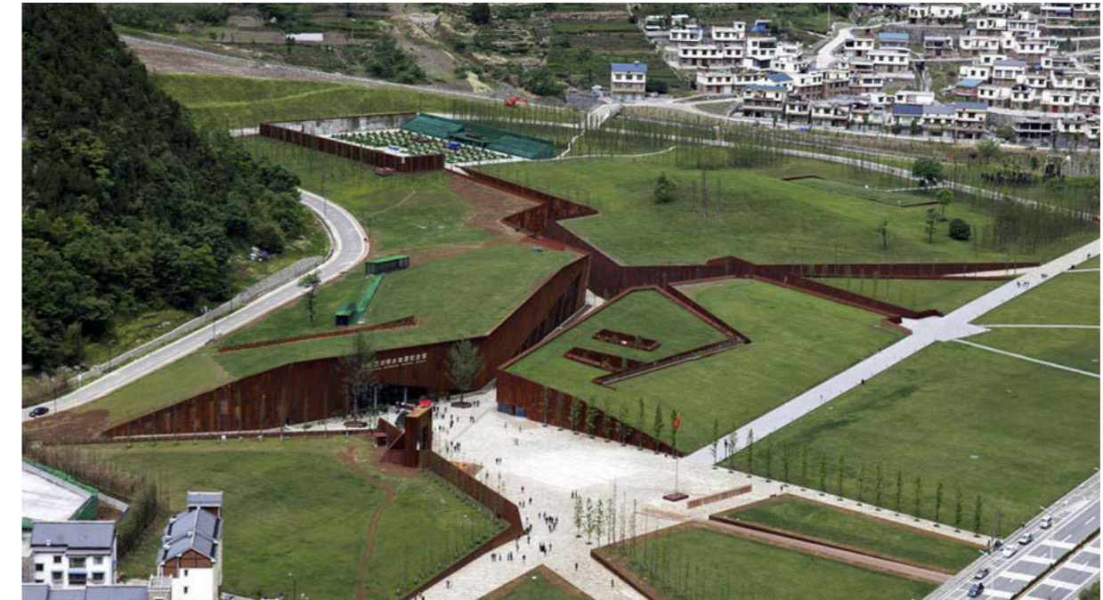
Image 2.88: The aerial photo of the Beichuan earthquake memorial gives you an idea of the crack landscape, 2013.
