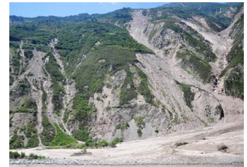
1.47: There are many landslid besides the Min river vally, caused by the Cascade hydroelectric station.
