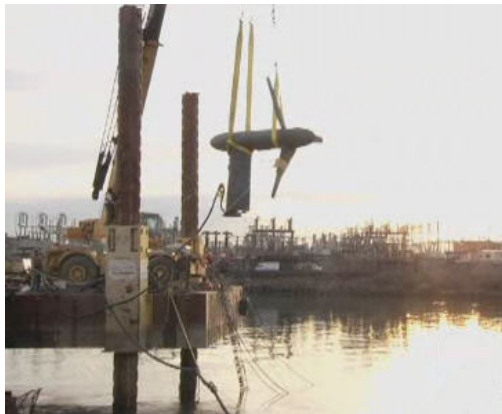
Figure 24: Experimental tidal turbine in Roosevelt Island, Manhattan
