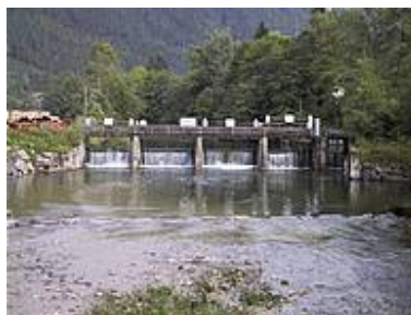
Figure 19: Small hydropower plant in Austria
