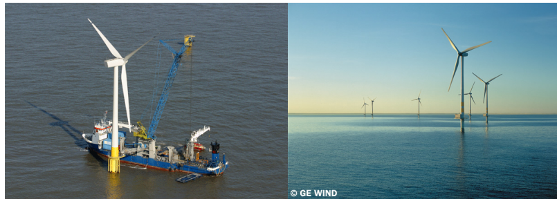
Figure 12: Off-shore wind turbine assembly and wind farm
