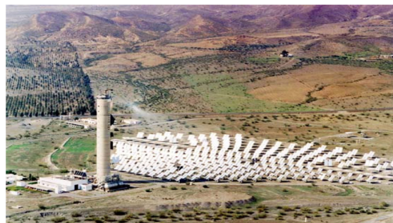
Figure 16: Solar Tower, diagram and experimental 7MW, Plataforma Solar de Almería, Spain
