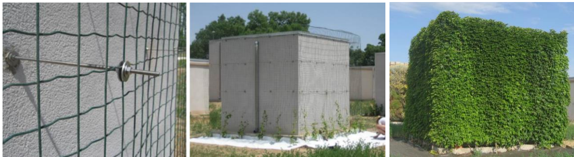
Figure 14. Double-skin green facade under study made with Boston Ivy ( Parthenocissus tricuspidata ), left, summer 2013; right, summer 2015
