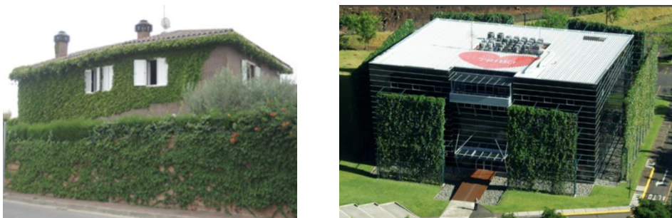
Figure 5. Left, traditional green facade in Lleida (Spain); right, double-skin green facade in Pergola building (Costa Rica), architect Bruno Santiago
