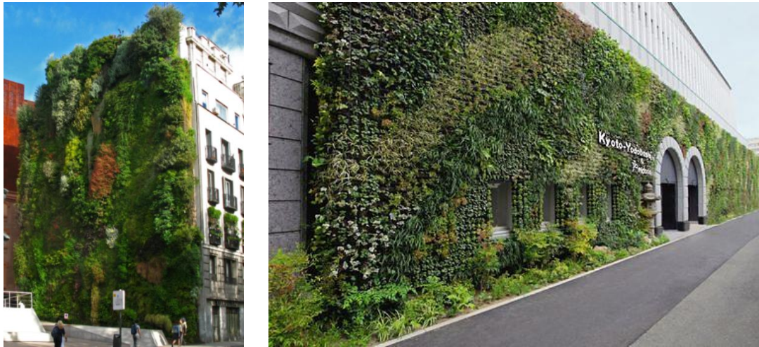
Figure 6. Green walls or living walls. Left, GW made of geotextile felt in Caixa Forum building, Madrid; right, GW made of panels in Multimedia Kyoto building (Japan), by Suntory Midory
