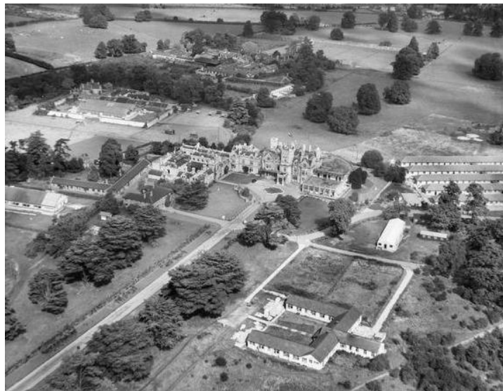
Figura 19. Preston Hall Sanatorium at the British Legion Village, Aylesford, 1919.
