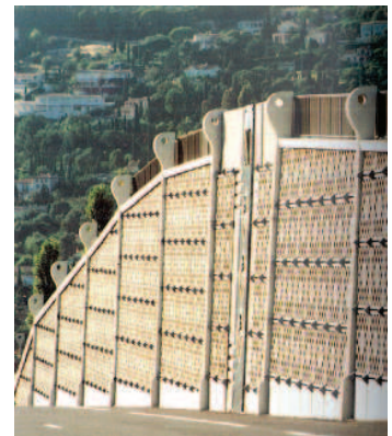
[s33] Cannes-Grasse Motorway, an example of one sided barrier.
