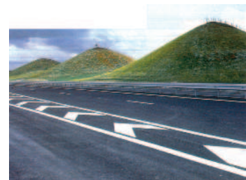
[s11] Troyes Rest Area. Depending on speed, the mounds perform as filter or screen.
