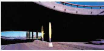
[s16] Interchange in Höfdabakka with a singular median.
