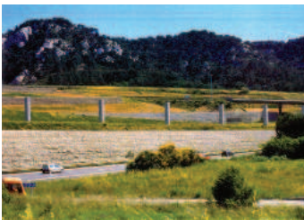
[s17] The design of the interchange makes directions more clear.
