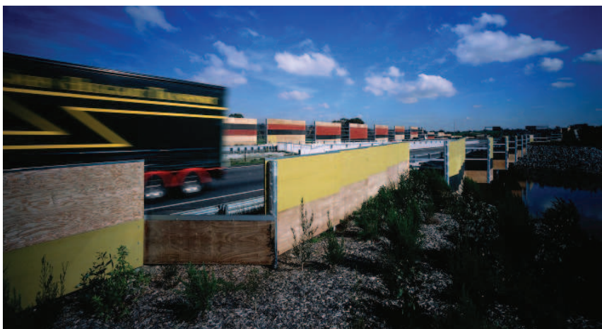
[s40] Monash Freeway Hallam Bypass.
