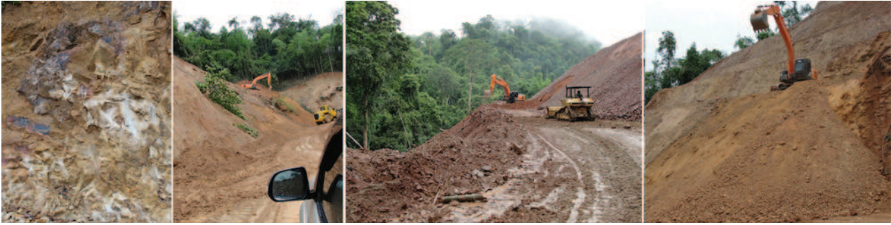
[12] The access road under construction.
