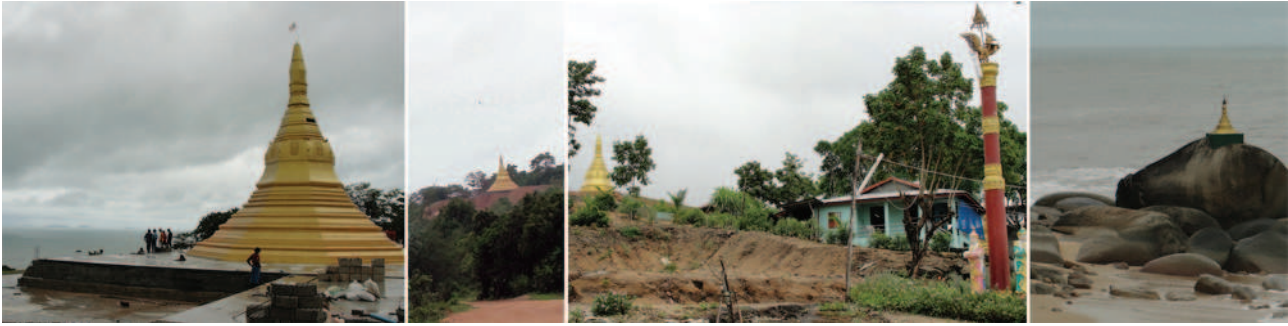
[3] Construction of Sule Potu Pagoda at Ma Yin Gyi beach by CSR and ITD construction team.
