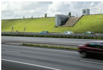
[s61] The slope to support artistic elements. Observatoire, Nieuw-Terbrugge.
