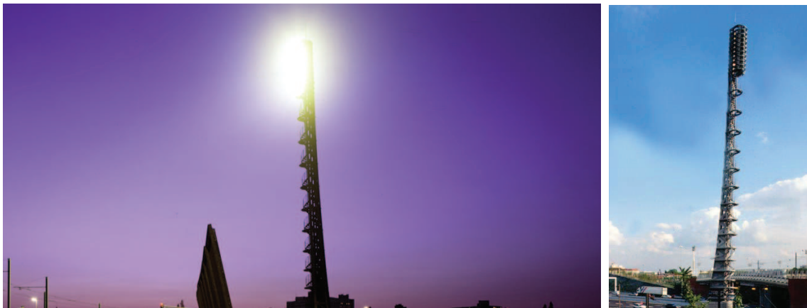
[s63] La Courneuve Light Tower.
