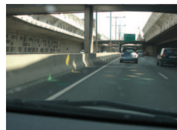
[s34] Acoustic barriers along Gran Via in Barcelona, a combination of a closed and linear sequence.
