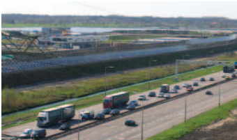
[s29] The acoustic barrier by ONL in Utrecht, a combination of apparent mobility and aerodynamic design.
