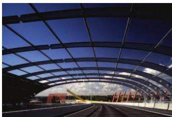
[s21] Falso túnel: Melbourne Gateway.
