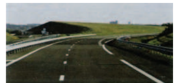
[s55] Use of the terrain and the vegetation to attenuate the tunnel effect of the more conventional cut and fill sections. Bernard Lassus.
