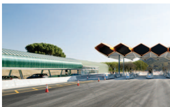
[s19] False cut section: the canopy of the service parking simulates a false slope. AP-7 Tolls.
