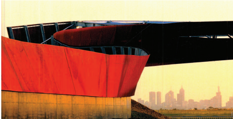
[s38] Craigieburn Bypass: Curtain Wall.
