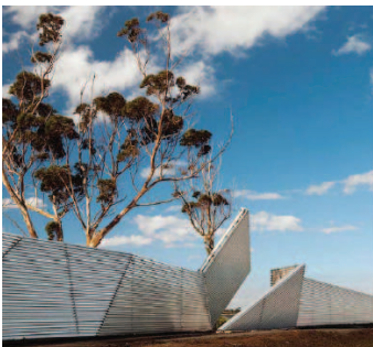
[s41] Textured noise barriers in the Deer Park Bypass.
