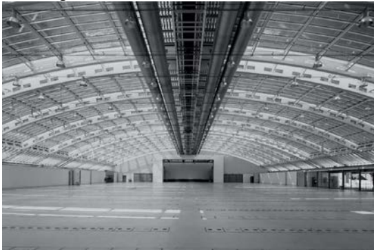
Figure 55: Design Center: exhibition hall with the ventilation system
