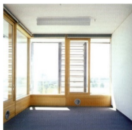
1 and 2 Office: inner facade layer with provision For natural and artificial ventilation; Air supply in apron wall
