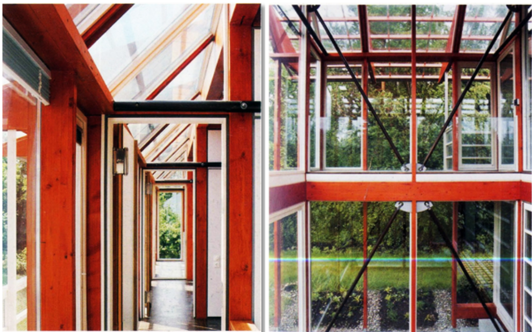
Figure 9: Two-family House, Pullach, Surrounding walkways at the upper levels
