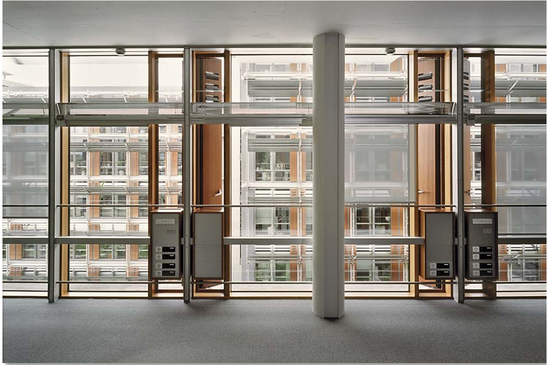
Frontal view of façade axis with the following components: vertical ventilation flap, open (left), closed (right). composed of a frame of laminated spruce, plywood with cherry mahogany veneer, insulation, integrated, adjustable ventilation flaps, lighting strip, wood box (left) with convector, wood box (right) with power supply.
