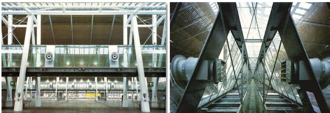
Figure 78: Hall 26, Hannover, Glass ventilation ducts
