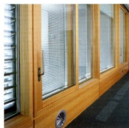
1 and 2 Office: inner facade layer with provision For natural and artificial ventilation; Air supply in apron wall
