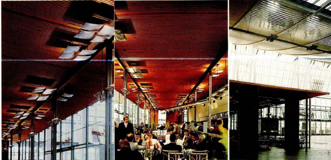
Figure 89: Hall 26, Hannover, Restaurant with soffit light-deflectors
