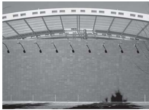
Figure 58: Design Center, end wall with the claytile facade
