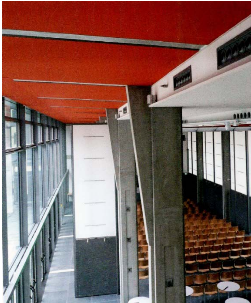
Figure 35: Oskar von Miller Forum, intelligent control systems which ensure automatic operations to meet the various needs within the building
