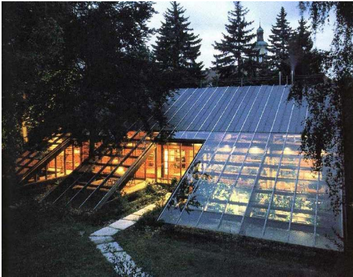
Figure 3: House in Regensburg, glazed southern face
