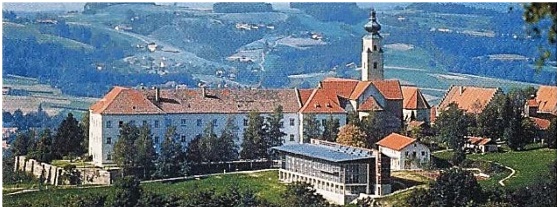
Figure 40: Aerial view, Guest Building for the Youth Educational Centre, Windberg
