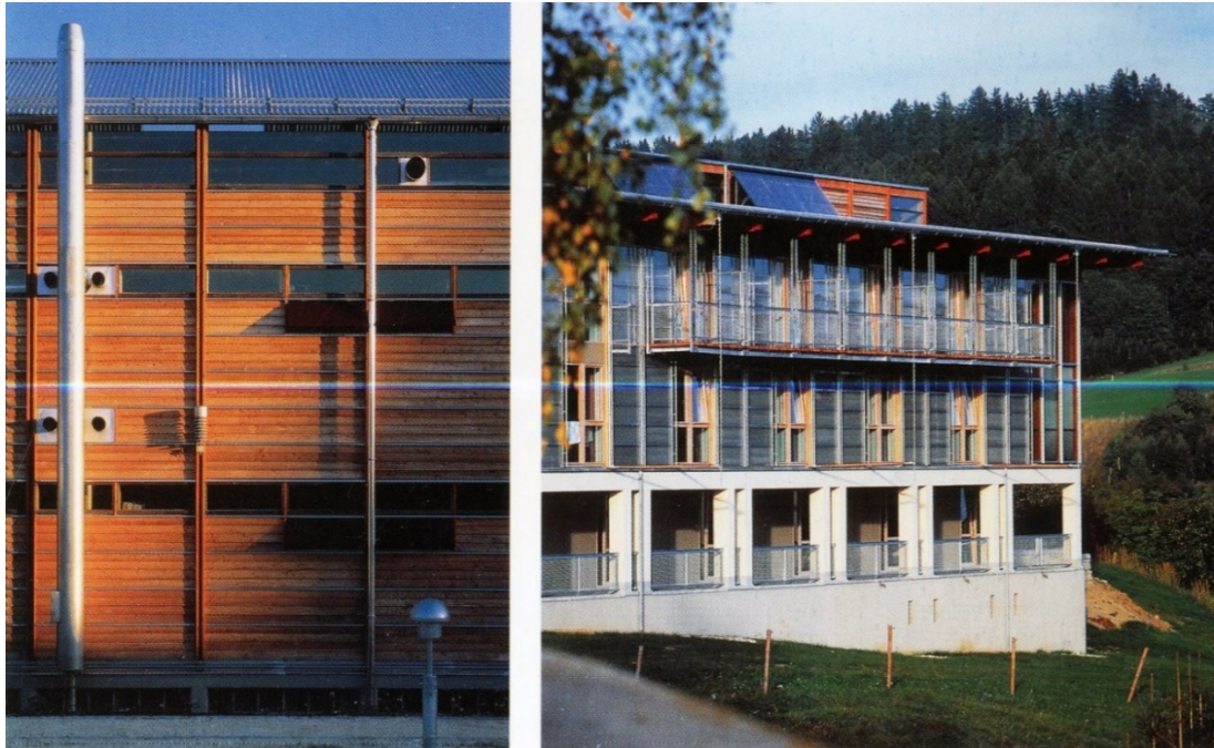
Figure 14: Guest Building, Windberg, Northern façade. Figure 15: Guest Building, Windberg, Southern façade.
