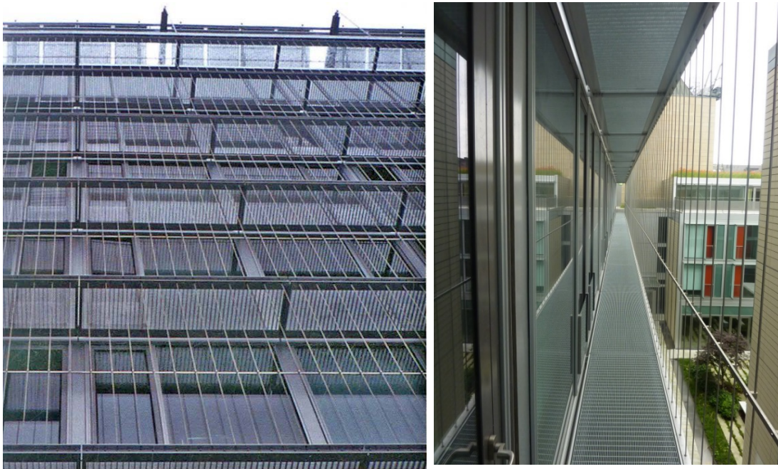
Figure 22: Oskar von Miller Forum, escape balconies and a series of vertical rods
