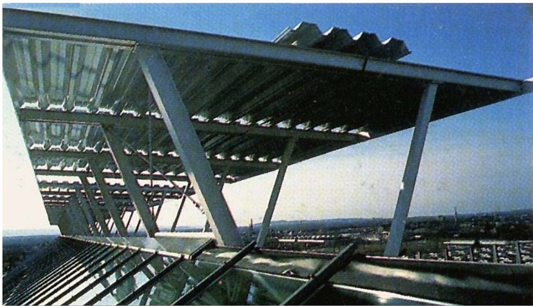
Figure 79: Hall 26, Hannover, "Venturi" capping over crest of roof
