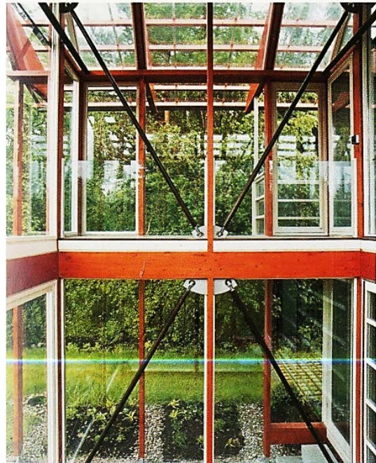
Figure 37: Two-family House, Pullach, Two-story conservatory space with wind Bracing
