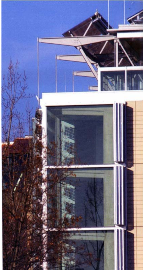
Figure 21: Oskar von Miller Forum, independent steel structure, over the south side
