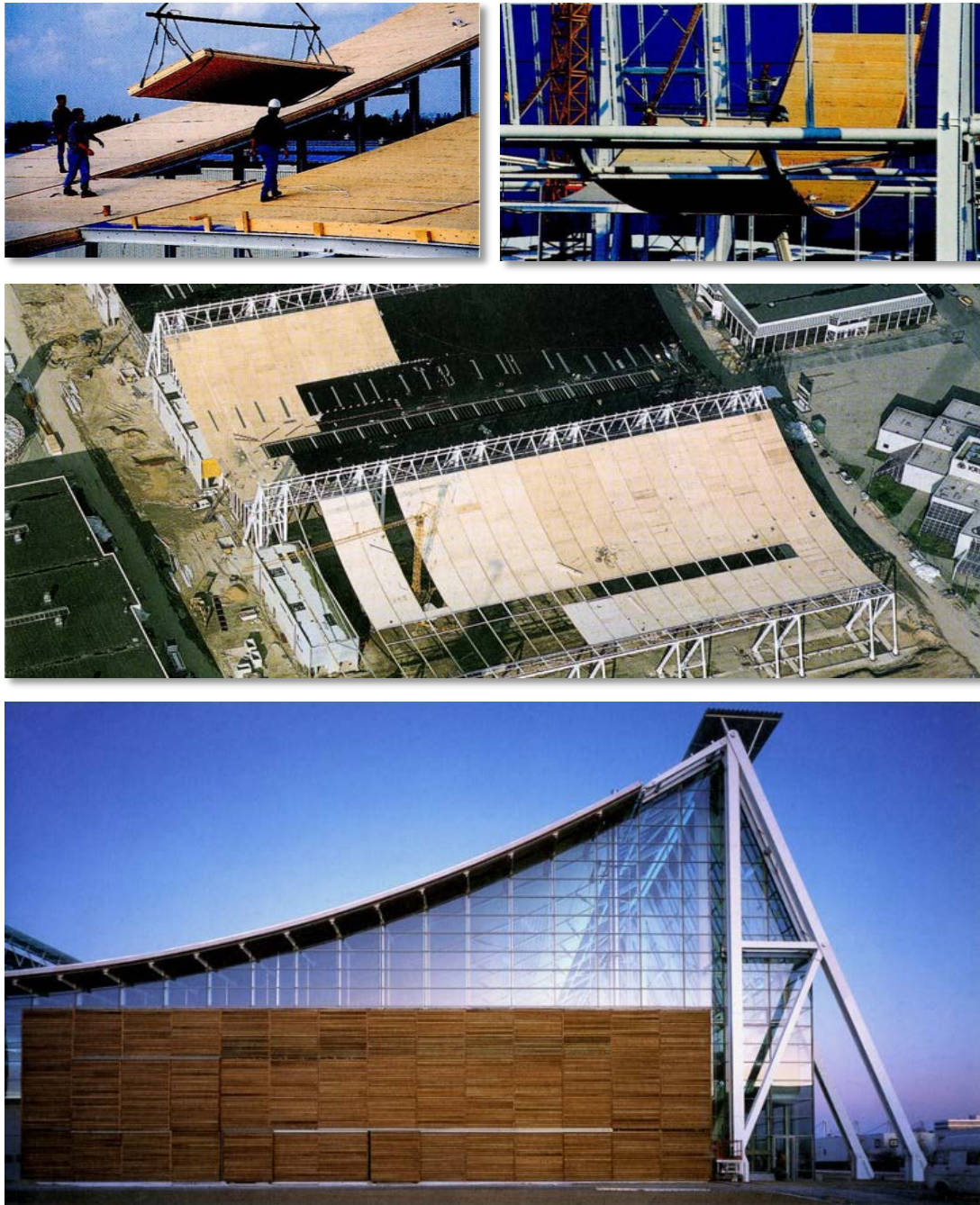
Figure 69: Hall 26, Hannover, Using timber as a renewable material
