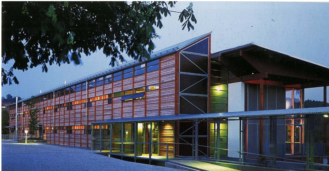
Figure 45: Guest Building, Windberg, Timber boarded front facing the village
