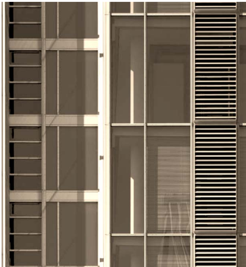
Figure 76: DMAG, double-skin facade with fixed glazing
