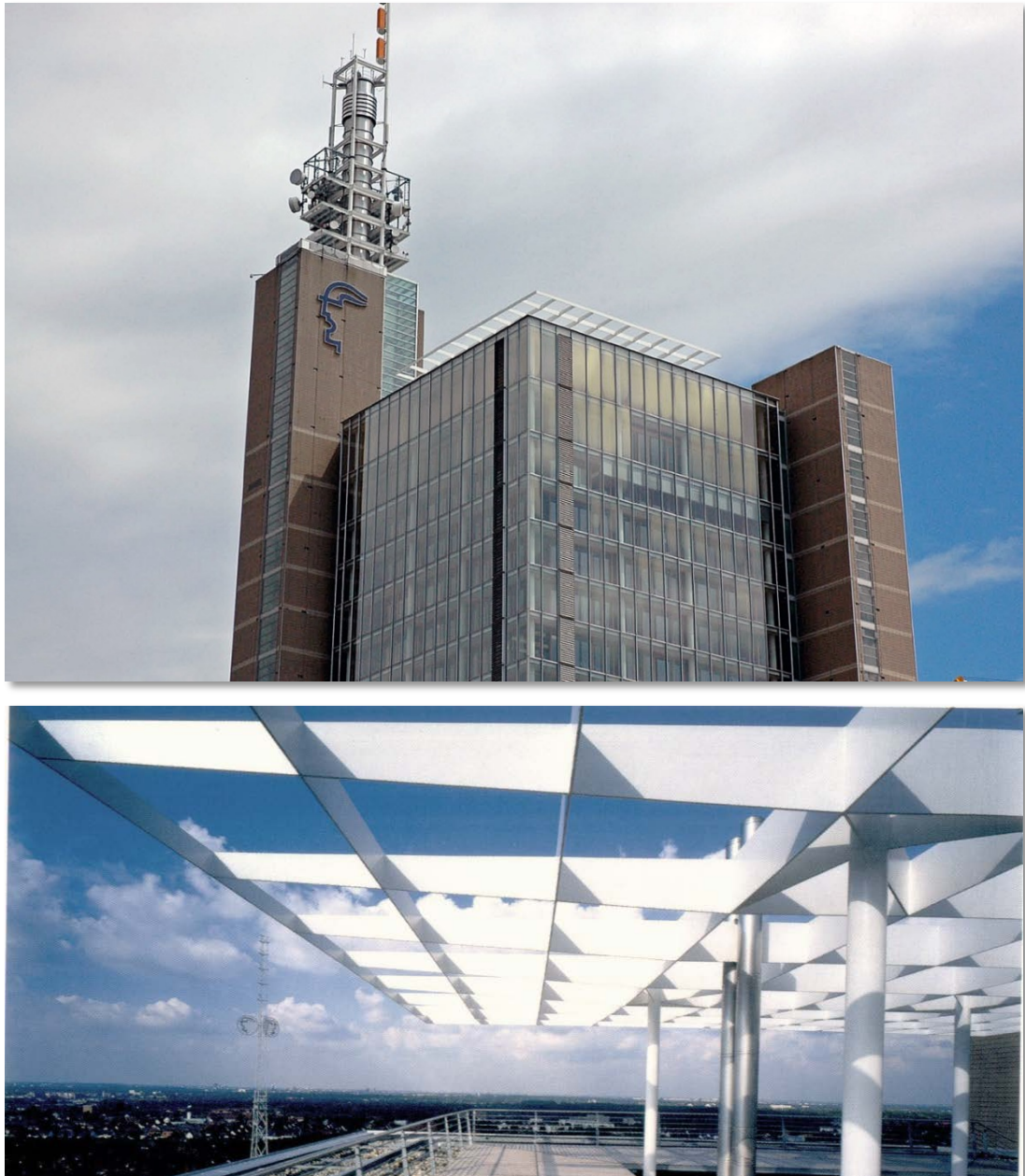
Figure 92: Administration building, Hannover, Roof level
