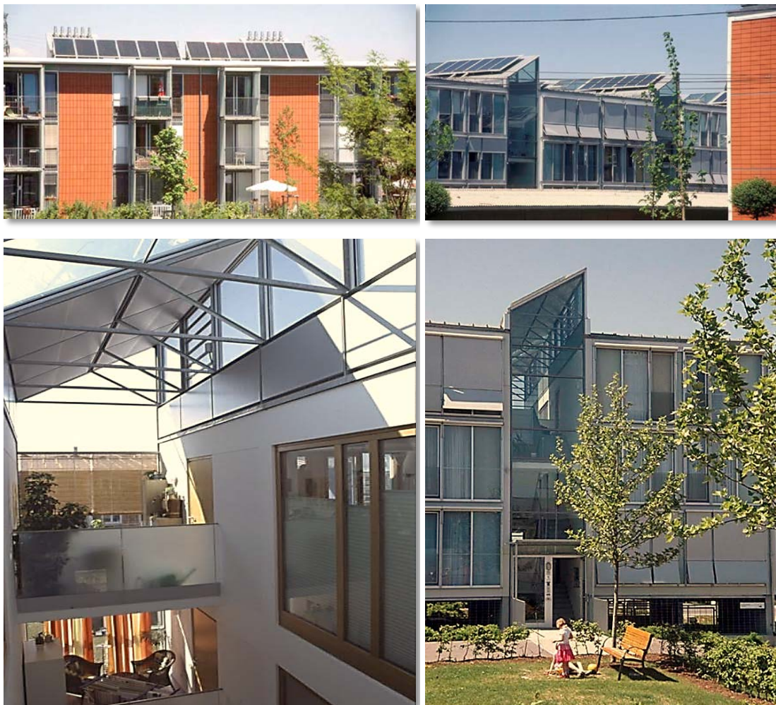
Figure 56: Solar city, Linz, PV collectors applied
