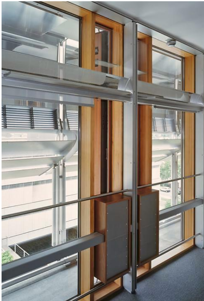
Figure 127: Office complex, Wiesbaden, Building technology installed on the facade
