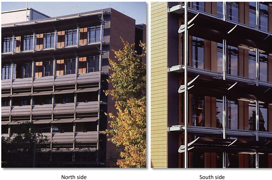
Figure 123: Office complex, Wiesbaden, North & South face
