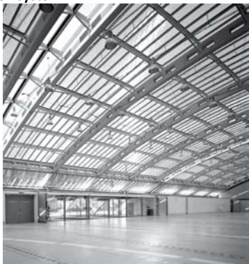
Figure 57: Design Centers, Steel girders framing the roof structure
