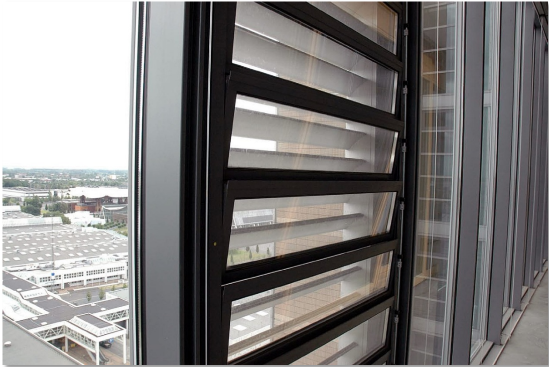
Figure 95: Administration building, Hannover, Adjustable glass louvers with automatic setting
