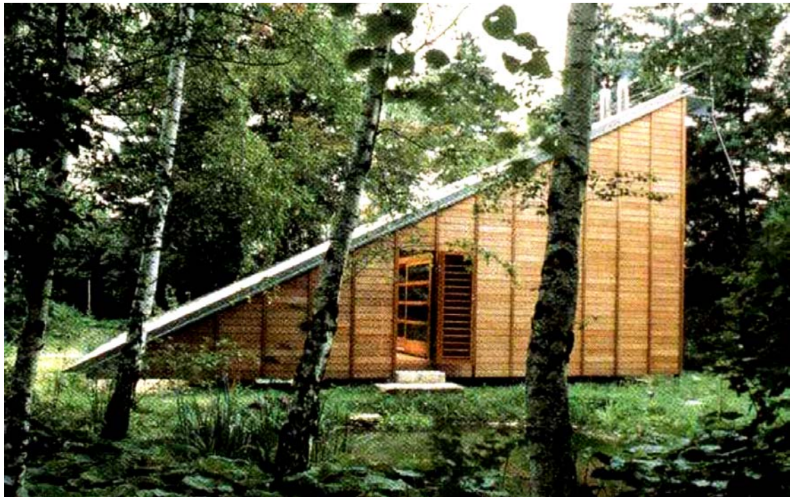
Figure 2: Thomas Herzog's 1977 House in Regensburg
