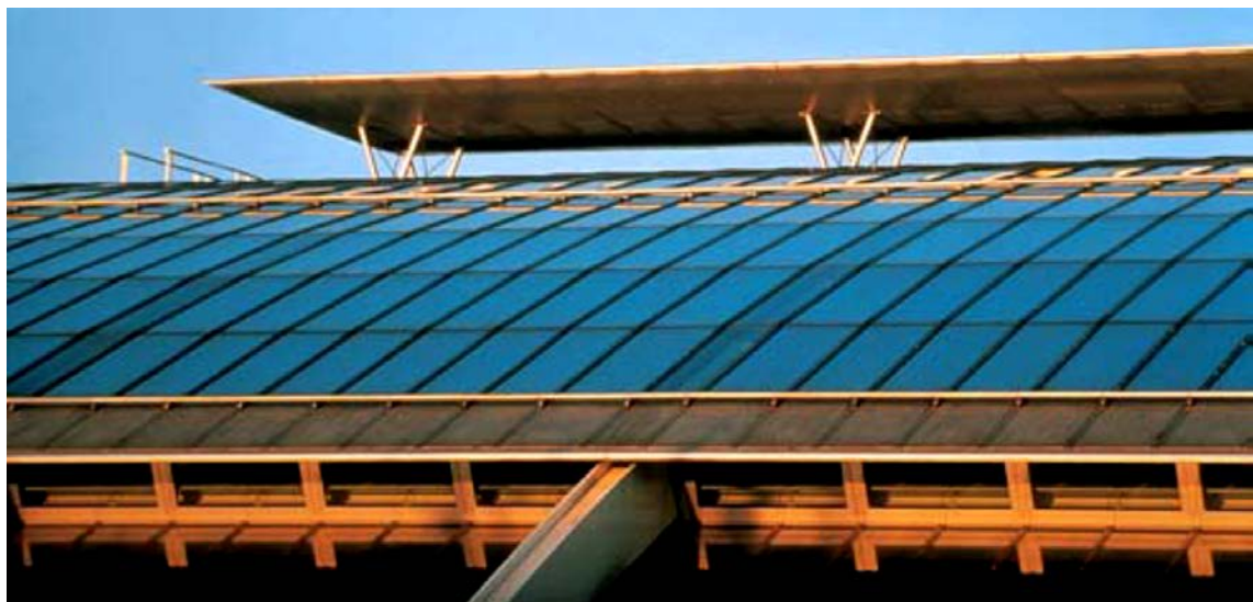
Figure 61: Design Center, long face of the hall with “Venturi” capping to assist natural ventilation
