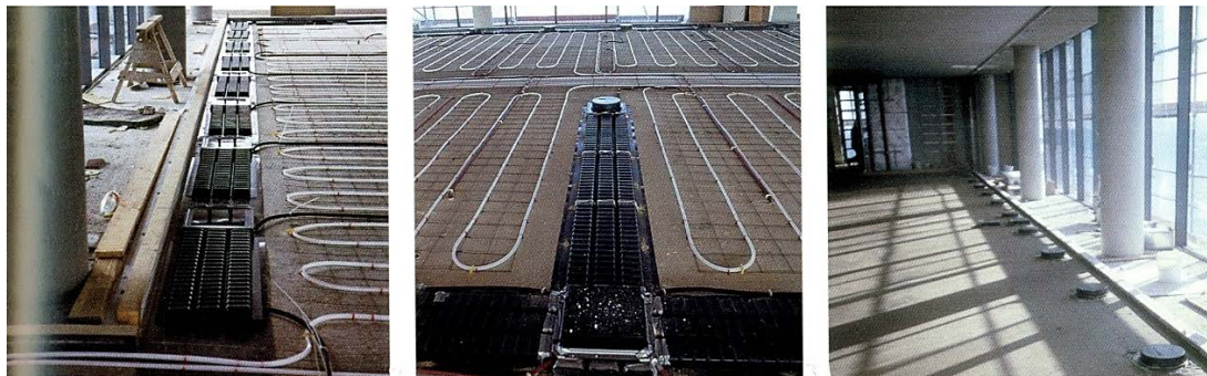
Figure 115: Administration building, Hannover, Thermoactive floor slab during construction
