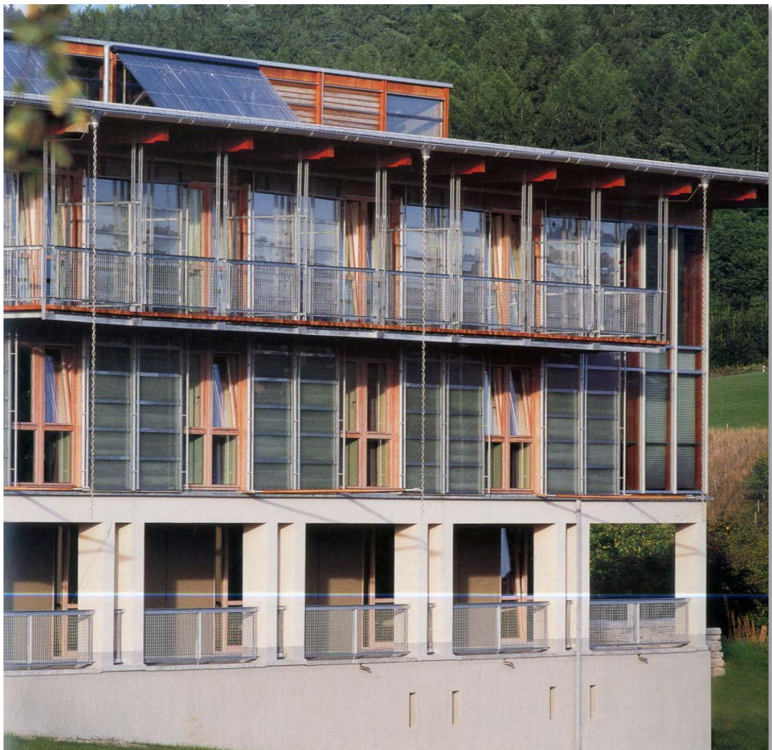
Figure 20: Guest Building, Windberg, south elevation with TIM elements in front of opaque wall element on upper two floors
