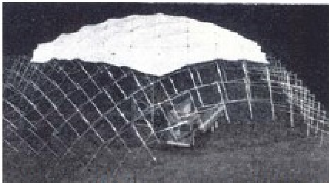
Working study model for a traveling deployable theatre (Emilio Pérez Piñero Foundation 2012).
