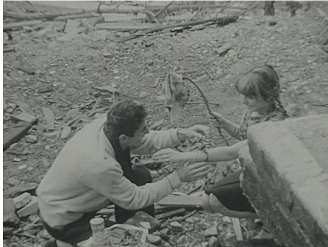
Figure 64. Rows of houses and home in the debris
