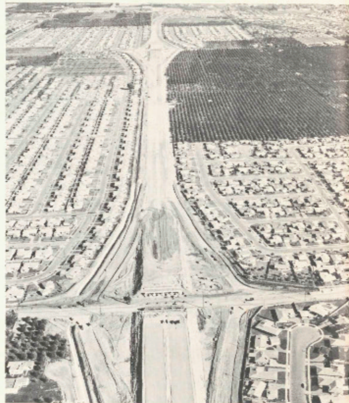
The right-of-way of this freeway in Riverside County, California, has been protected by subdivision controls which insured that the future residential developments would fit in with the highway plan.
