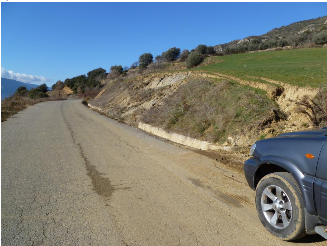
Figure 3-9: Slide material. Fine colluvium from the Upper Red Garumnian (Photo: Guillem Domènech).
