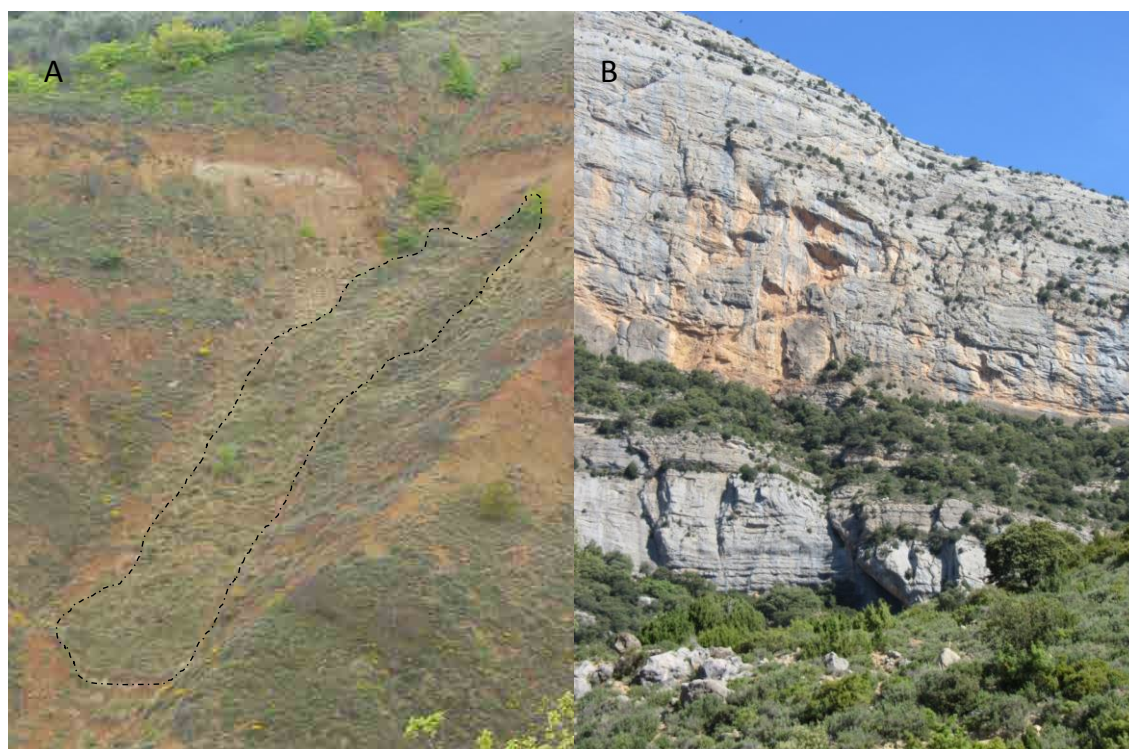
Figure 2-6: A) Earthflow at the Barcedana Valley in Garumnian materials. B) Rockfalls occurrences in the Upper Cretaceous limestones
