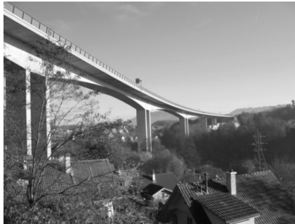
Figure 2.11 Overview of Felsenau viaduct(Zogg and Ingensand 2008).
