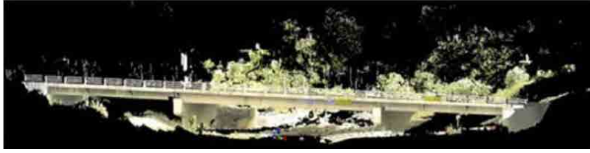
Figure 2.14 Coarse scan from Station 1 for the bridge(Mosalam, Takhirov et al. 2014).
