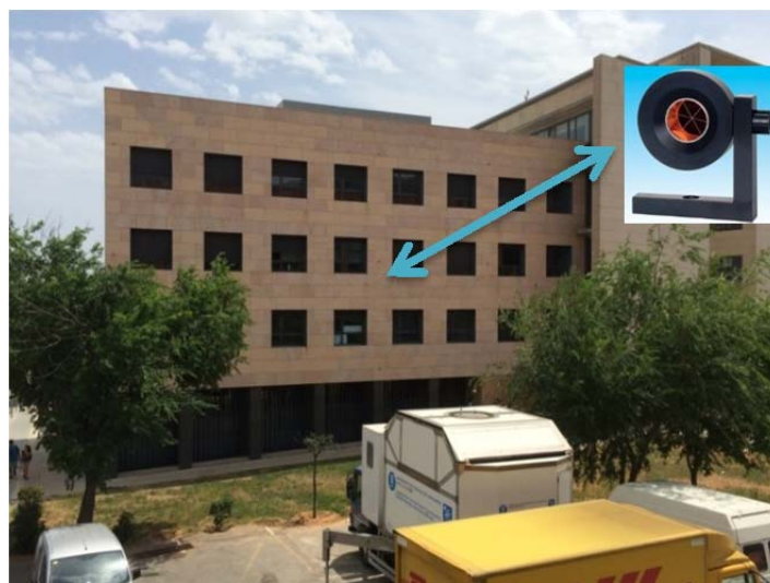
Figure 4.4 Prisms on the K2M building.
