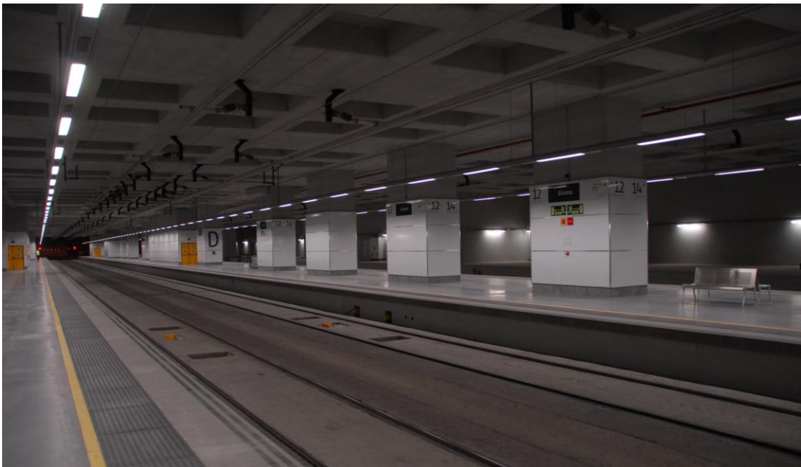
Figure 7.10. Picture of the station platform just after its full completion.
