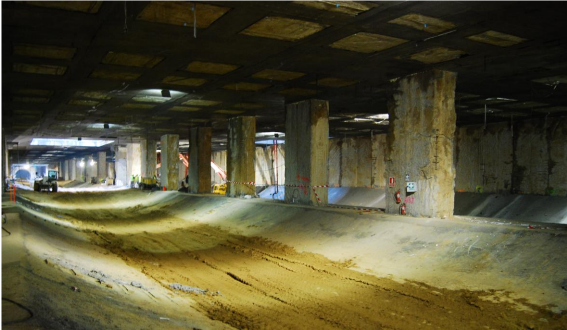
Figure 7.9. Picture of the station platform just before its full completion.
