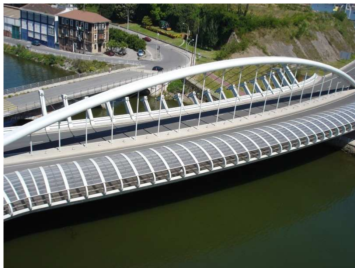
Figure 2-2: Bridge over Galindo river in Bilbao
