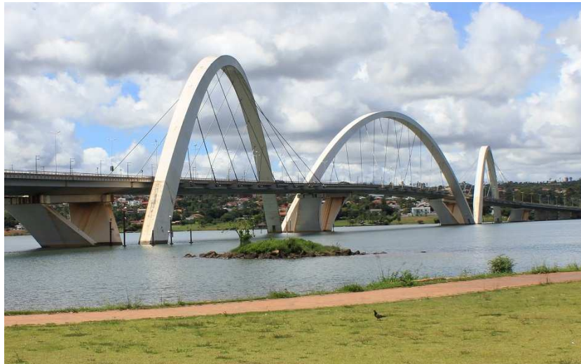
Figure 5-3: Juscelino Kubitschek bridge in Brasilia, over the lake Paranoá, Brazil, 2000-2002. Three arches rotated according to a vertical axis. (Reproduced by kind permission of Lukas Kohler). See Annex N1 for further details.
