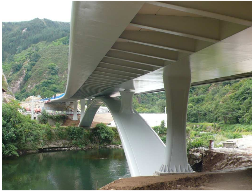
Figure 5-5: Enderlatsa bridge (Reproduced by permission of Javier Manterola). See Annex N1 for further details.
