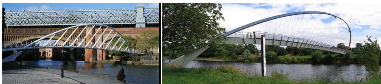
(a) (b) Figure 2-8: (a) Merchants Bridge. (b) York Millenium Bridge
