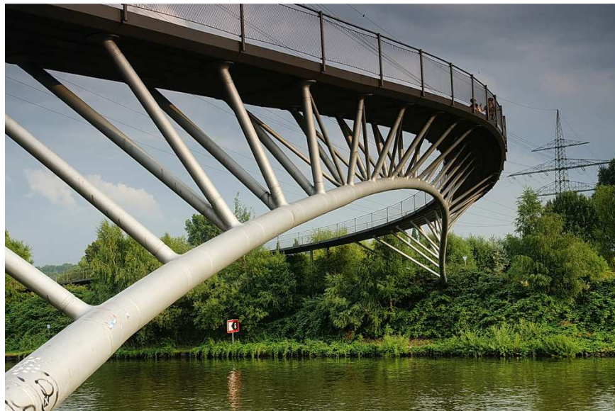
Figure 5-4: Ripshorst bridge (Reproduced by kind permission of Mike Schlaich). See Annex N1 for further details.
