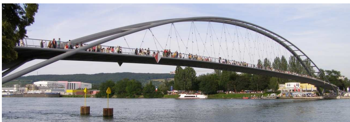
Figure 2-9: Dreiländer bridge (reproduced by kind permission of Hans-Peter Andrä)
