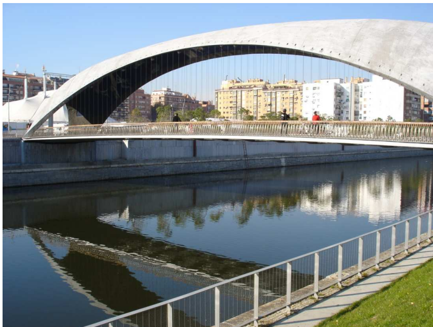
Figure 5-6: Invernadero footbridge. See Annex N1 for further details.
