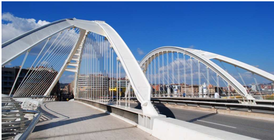
Figure 5-2: Bac de Roda bridge (see Annex N1 for further details)
