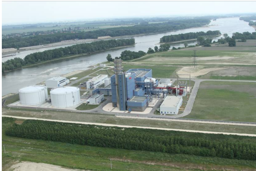
Figure 8-14: 430 MW CCGT power plant in Gönyü (Hungary) at river Danube 1
