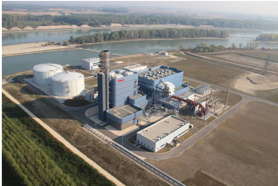
Figure 7-1: 400 MW CCGT Power Plant in Gönyü (Hungary) at river Danube
