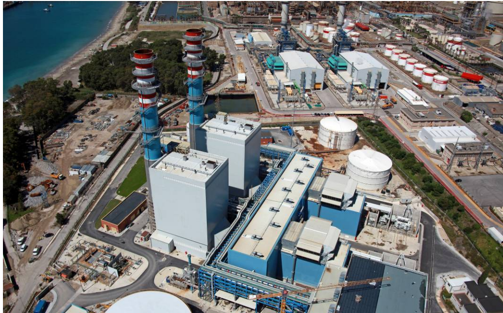
Figure 6-7 : Two CCGT Power Plants, each with two gas turbines in Algeciras (Spain)
