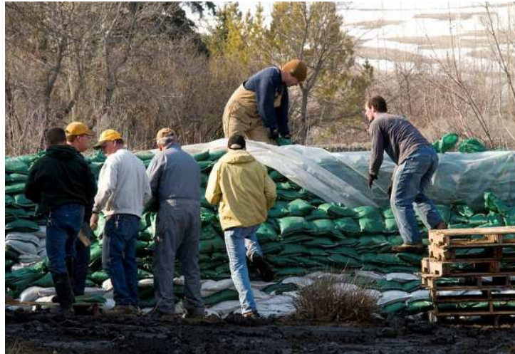
Figure 1.7 Valley City neighbourhood use sandbags to create a levee along the Sheyenne River (by Patsy Lynch/FEMA)
