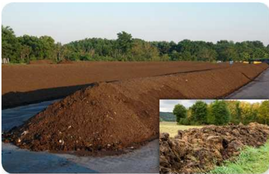
Figure 1.1: Composting process (windrow) of contaminated soil.
