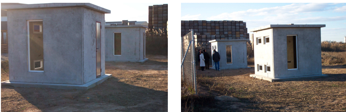
Figure 55. View of the concrete cubicles (2006).
