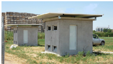
Figure 57. View of the cubicles with awning; July 30 th , 2008 at 13:30 pm.
