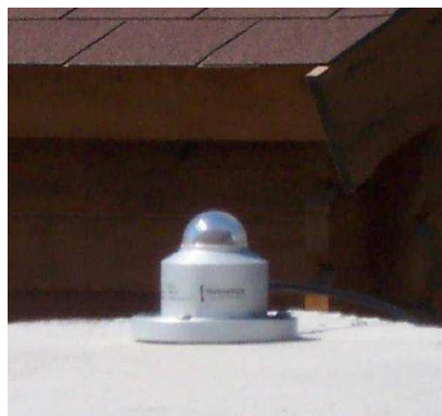
Figure 61. Solarimeter placed on top of the cubicles.
