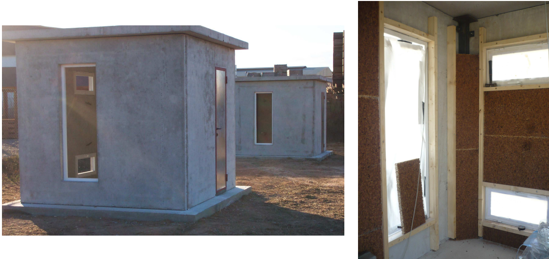
Figure 145. Current view of the concrete cubicles: outer view (left), and inner view with the interchangeable inner insulation and plasterboard (right).
