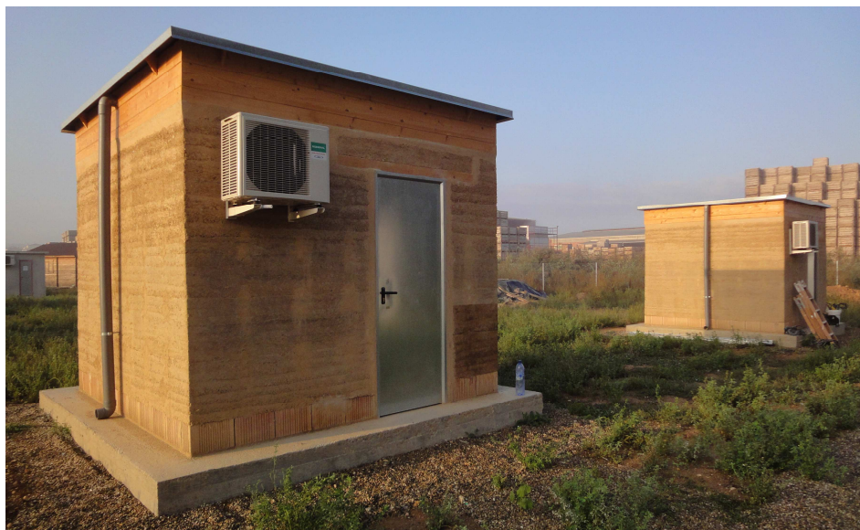
Figure 149. Outer view of the rammed earth cubicles.
