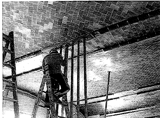
Figure 5.11 –Props supporting the Lower vault.
