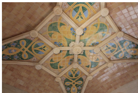
Figure 5.9 – One of the intermediate vaults, Administration building.
