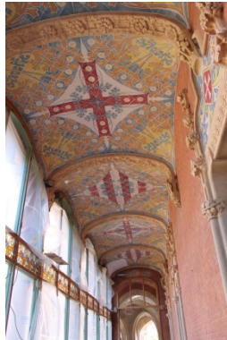
Figure 5.8 – Small vaults in a row, Administration building.
