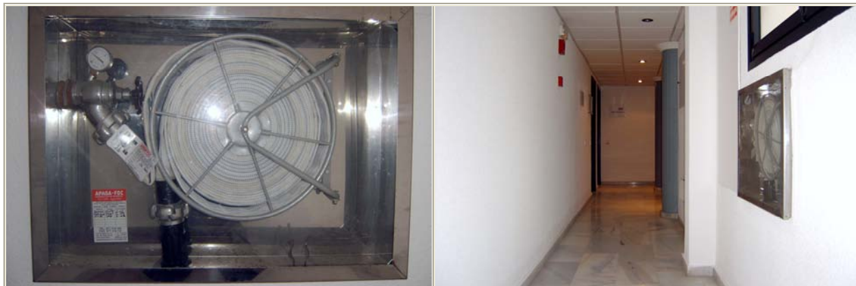
Figure 6-32. Photographs of the hose-nozzle employed by the fire-fighter.
