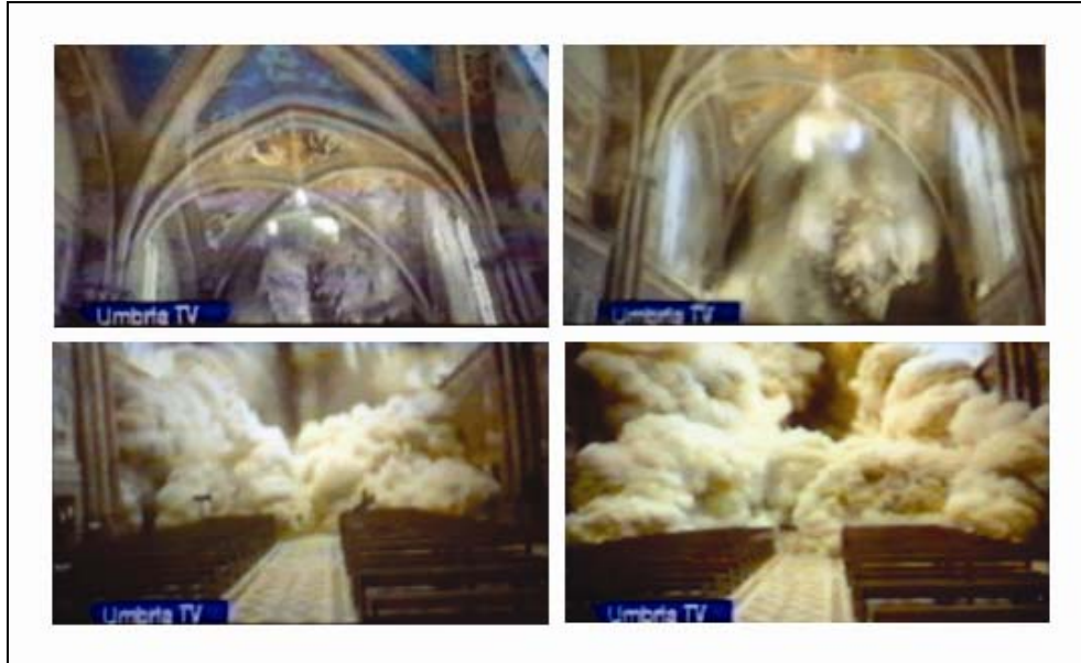
Figure 1.1 Photo sequence of the transept vault partial collapse occurred in the Basilica of Saint Francis in Assisi, Italy, during the Umbria-Marche earthquake (1997).
