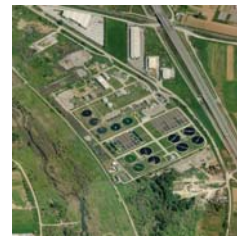
G. treatment plant
