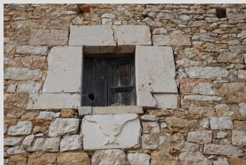
Fig. 21 Ventana fachada principal
