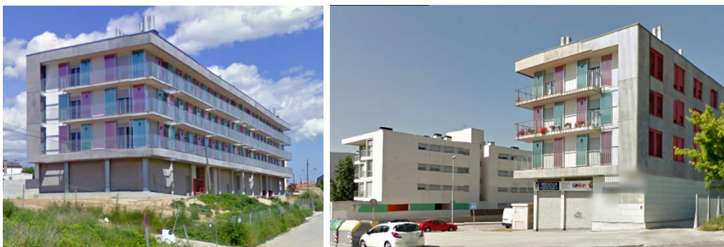
Figure 5.2. Photos of the building from south-west and north-east (adapted from www.google.com [2014 05 21]).
