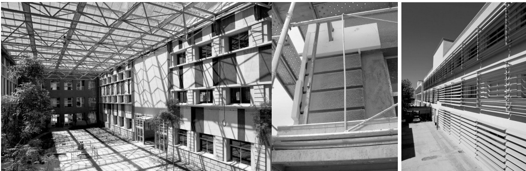
Figure 2: Gardeny office buildings. Inner view of the patio once they are covered by the glass green house structure, detail of the isolation layer and details of the solar shadings devices
