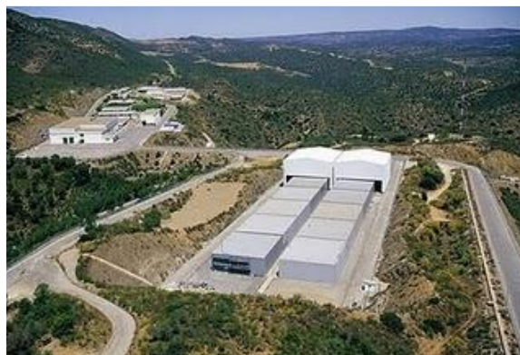
Figure 1.1. El Cabril disposal facility.
