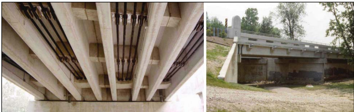
Figure 2.14. First traffic bridge with CFRP tendons built in United States [111,112].
