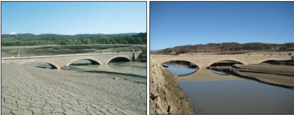
Figure 1.3. Evolution of the siltation in the Barasona Reservoir. Images illustrate the changes at the same section between September 2001 (left) and November 2007 (right). Left image was taken by Ramon J. Batalla in 2001.
