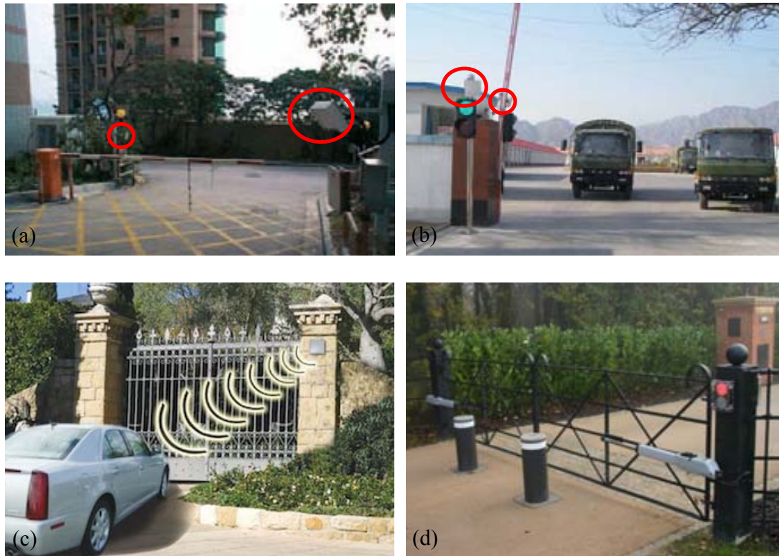
Fig. 5.8 Examples of AVI systems for (a) hospital access control, (b) access control of trucks, (c) access control in gated communities, and (d) area controlled by hydraulic rising bollards.
