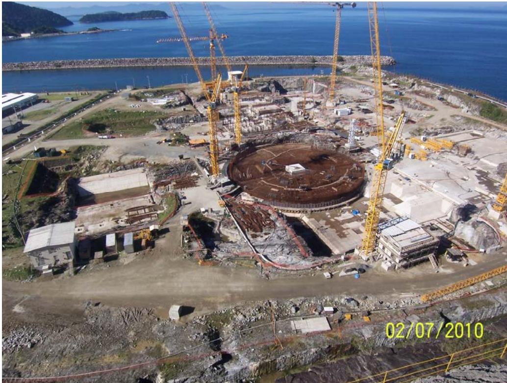
Fig.54: UNA3 foundation works as per July 2010 (Source: www.eletronuclear.gov.br ).
