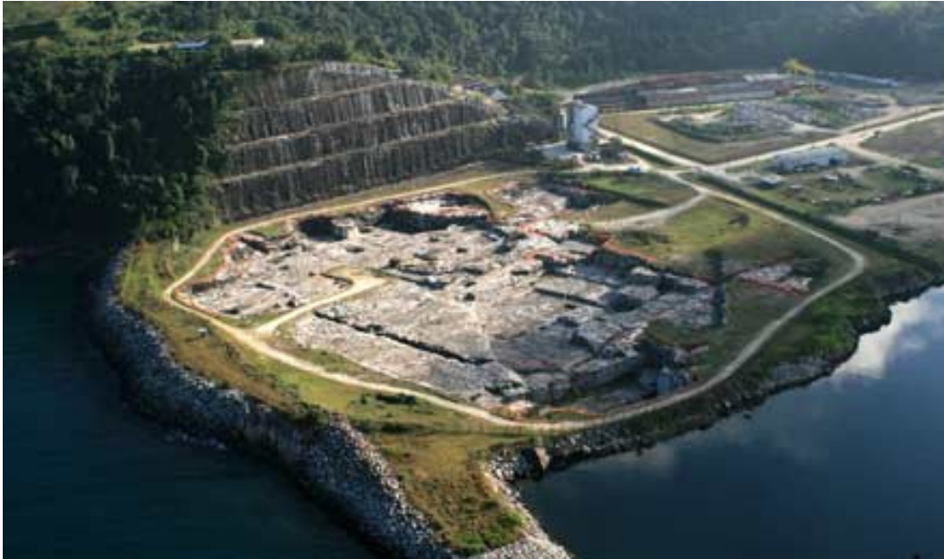
Fig.51: UNA3 initial earthworks as per April 1986 (Source: www.eletronuclear.gov.br )
