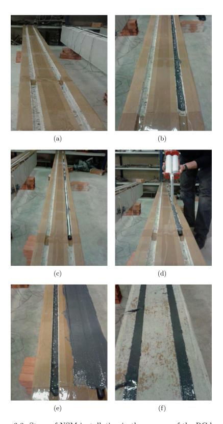
Figure 6.6: Steps of NSM installation in the grooves of the RC beams.
