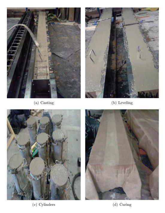
Figure 6.3: Procedure of casting and curing for beams and cylinders.
