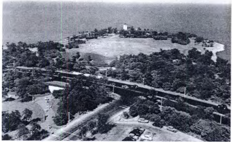
46. Alfred Caldwell. Promontory Point, Burnham Park, Hyde Park, Chicago, Illinois, 1936-1937. Vista desde los Promontory Apartments. Foto de 1946.
