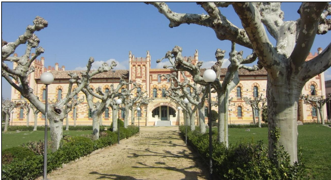
Figure 4.6. Vichy Catalán bathhouse designed by Gaietà Buigas following a Neo-Moorish style.
