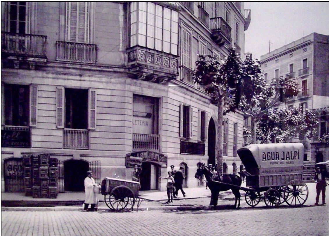
Figure 6.25. Jalpi water distribution centre in Barcelona.
