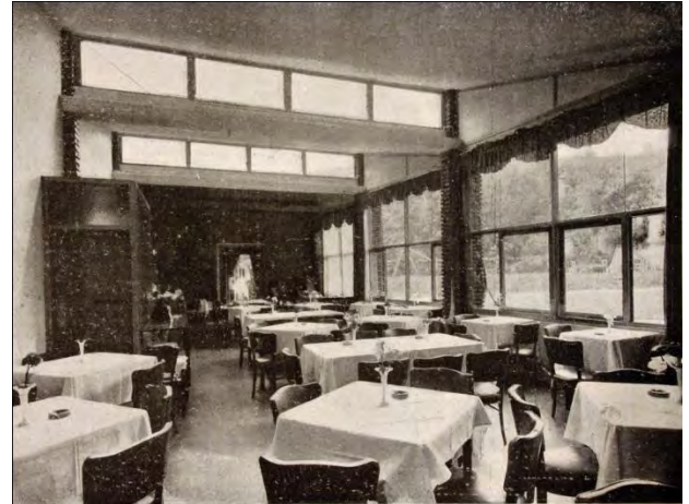
III.4.29 Vista interior del restaurant.
