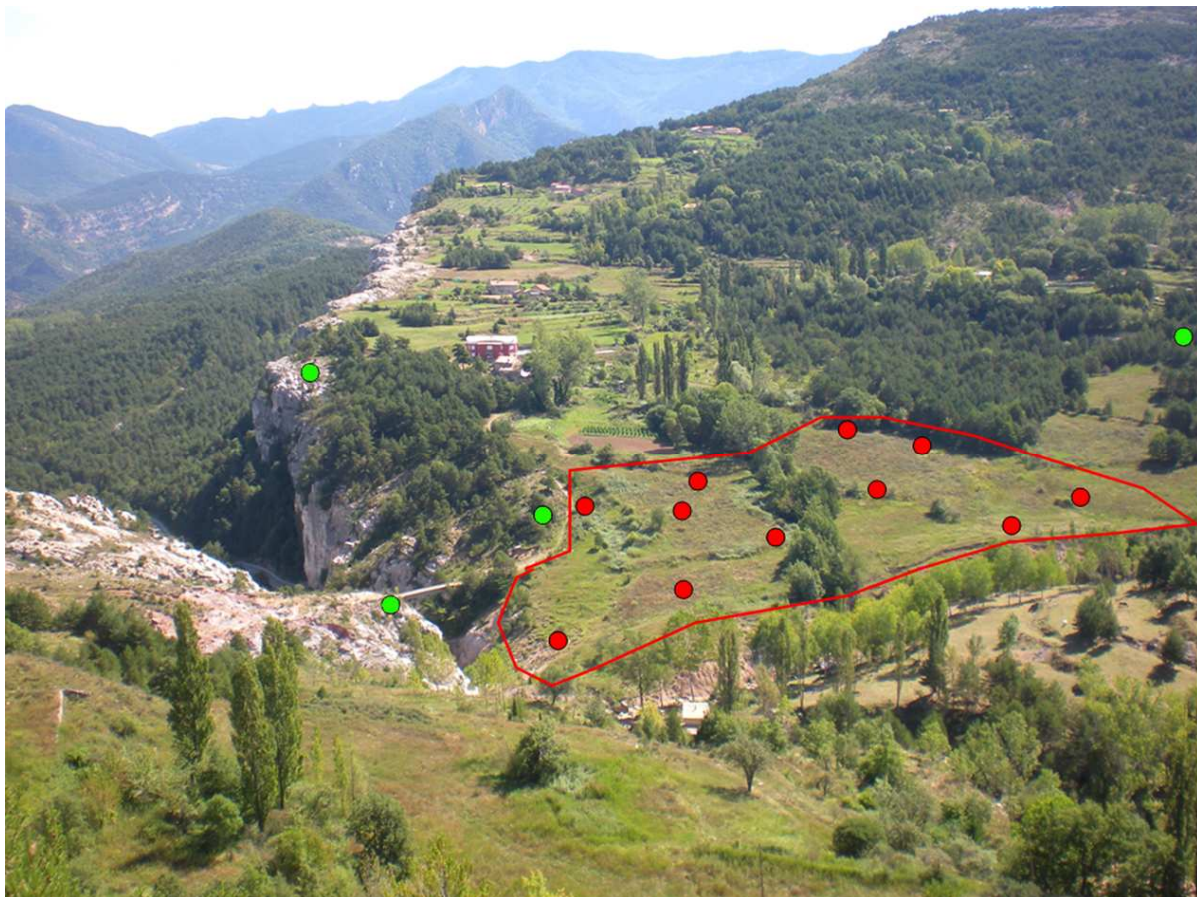
Figure 5.12: Vallcebre test site. The green points represent the stable CRs while the red ones represent the CR deployed on the area of movement.
