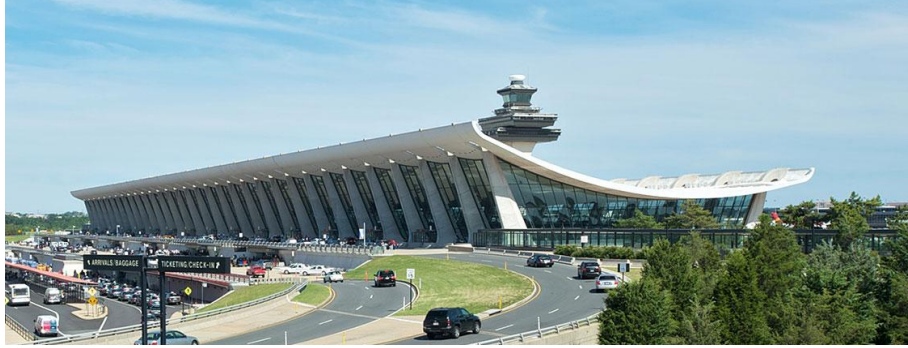
(a) The roof of the Dulles International Airport was designed by Eero Saarinen as a catenary.
