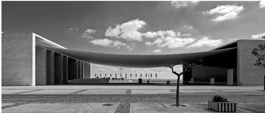
(d) The canopy of the Portuguese pavilion for the Expo'98 in Lisbon is a spectacular catenary conceived by Alvaro Siza Vieira and designed by Cecil Balmond.
