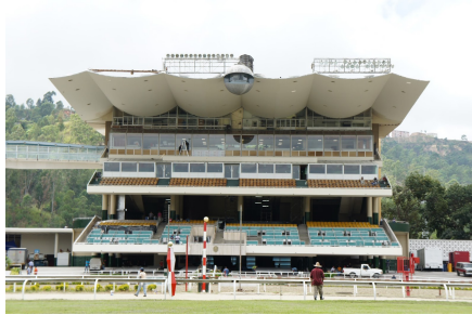
(b) The roof of the Caracas hipodrome was designed by Arthur Froehlich as a series of catenaries.
