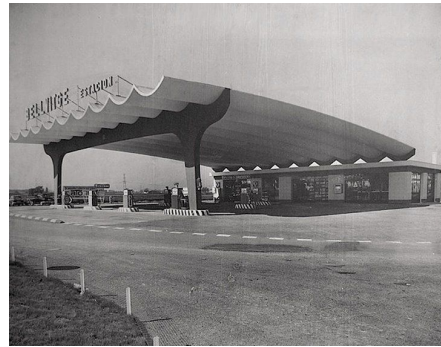
(c) The canopy of the Bellvitge gas station (Barcelona) was also designed as a series of catenaries.
