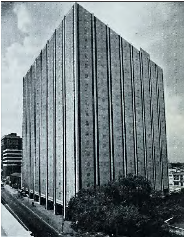
The Atlanta Merchandise Mart in 1961, before any of the other Peachtree center buildings had been constructed. The mart has since been enlarged twice the size shown, an expansion that had been provided for in the original plans.
