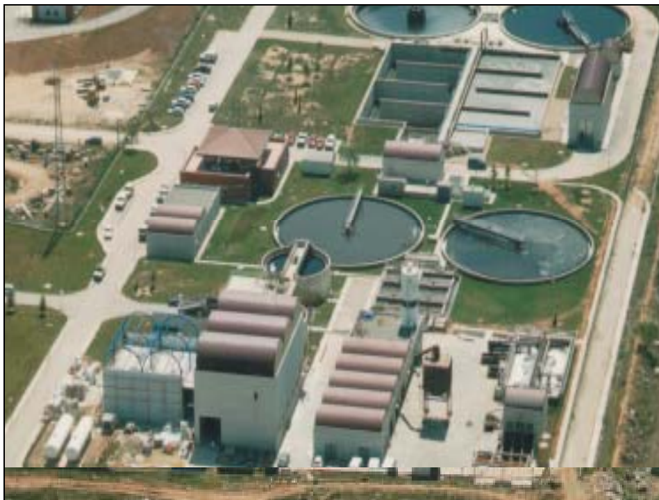
Figure 3-7: Picture of Granollers WWTP.
