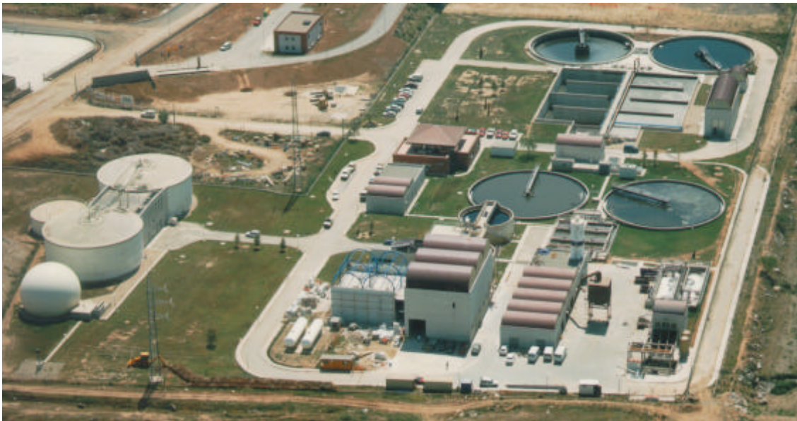
Picture 1 Aerial picture of the Granollers WWTP
