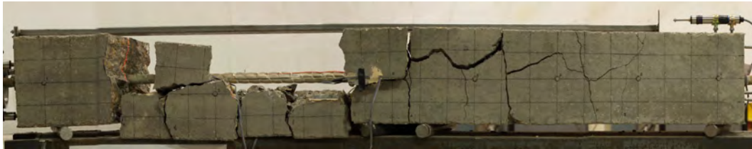
Figure B.14: Image final crack pattern (tie 19-170).
