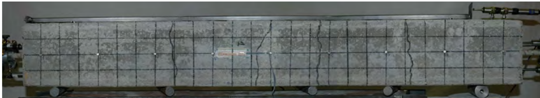
Figure B.6: Image final crack pattern (tie 16-170).
