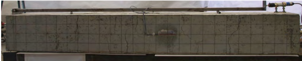
Figure B.18: Image final crack pattern (tie 16-170-2).
