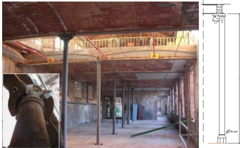
Figure 3.31 - Position and dimensions of the cast-iron pillars located at the ground floor of an existing masonry building in the Eixample district (Cornadó Bardón, 2015).
