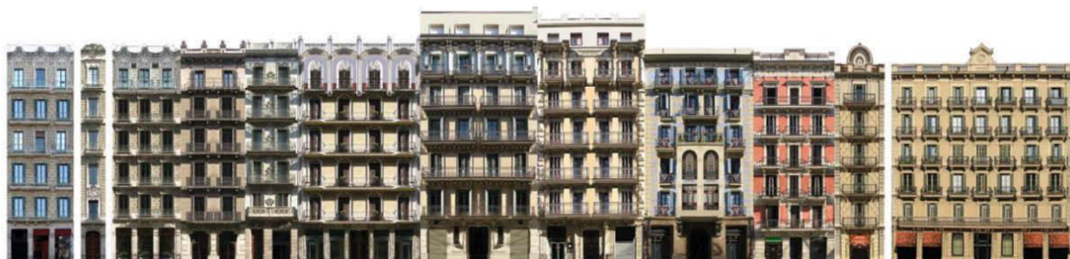
Figure 4.9 - Presence of staggered floors in a row of buildings in a typical example urban block (Castilla Marne, 2010).
