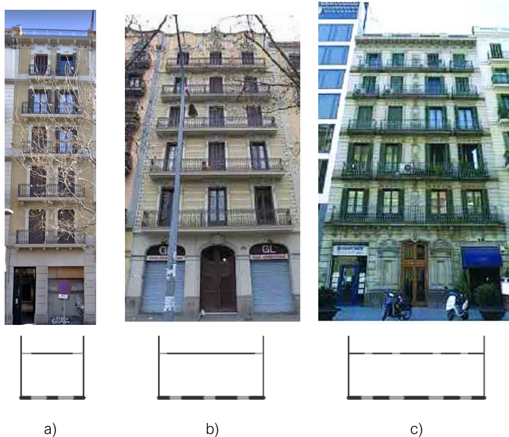
Figure 4.7 - Different number of façade openings on the ground floor and the upper levels: a) narrow building with two openings on the ground floor and each of the upper levels; b) band building with three openings at the ground floor and three on each floor level; c) band building with three openings at the ground floor and four on each floor level. The drawings represent the number of opening on the upper floor levels depending on the width of the façade (Cornadó Bardón, 2015).
