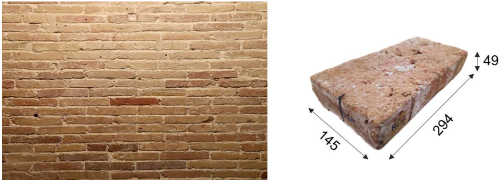
Figure 3.22 - Front view of a traditional solid brick masonry wall in an existing building in the Eixample district (left) and a solid brick unit with dimensions 294 x 145 x 49 mm (right).
