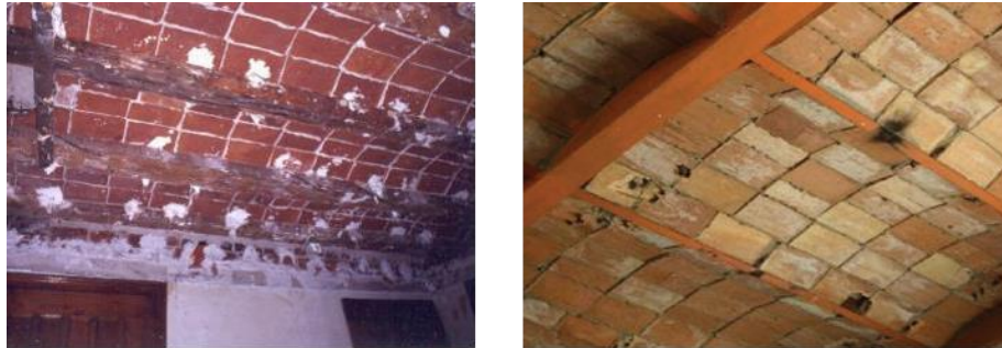
Figure 3.25 - Typical one-way flooring system with timber beams (left) or steel beams (right) and masonry vaults with flat ceramic tiles (Casanovas, Graus i Rovira, and Rosell 1993).
