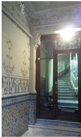
Figure 3.29 - Presence of masonry columns (" pilastres ") at the ground floor entrance of an existing masonry building in Eixample (Cornadó Bardón, 2015).
