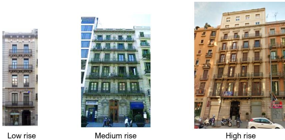
Figure 4.3 - Different height levels of existing masonry buildings in the Eixample district.
