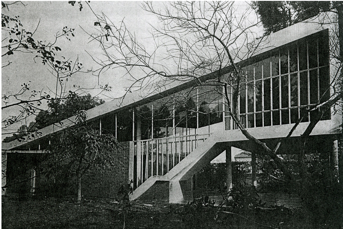
JOAO VILANOVA ARTIGAS RESIDENCIA PROPIA 1948, SAO PAULO, BRASIL Mindlin, Modern architecture in Brazil
