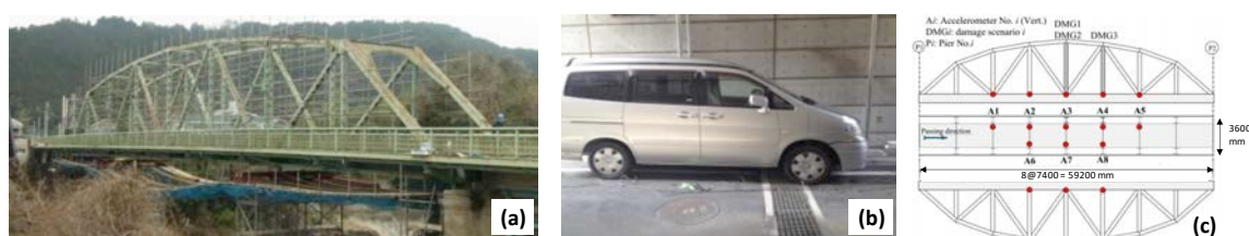
Figure 2. Illustration of (a) the Warren truss bridge (b) recreation vehicle used in the test (c) location of the 8 accelerometers and artificial damages. Adapted from reference 47 .
