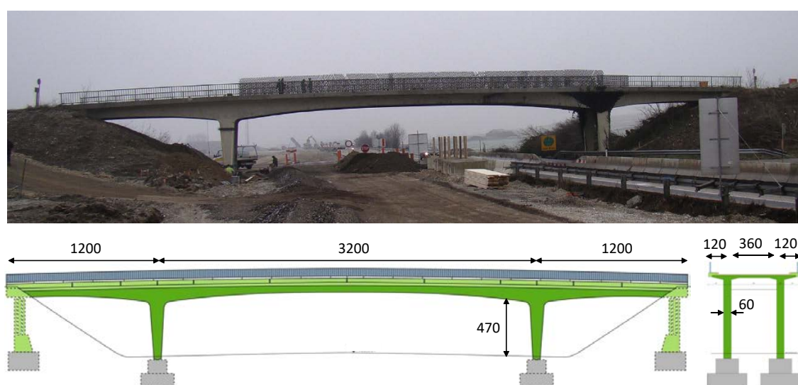
Figure 2. View of the S101 Bridge and bridge dimension (dimensions in centimeters)
