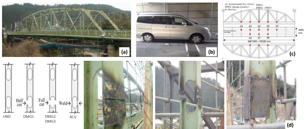
Figure 4.3. Illustration of (a) the Warren truss bridge (b) recreation vehicle used in the test (c) location of the 8 accelerometers and artificial damages (d) experimental programme of the artificial damage. [Adapted from reference 147].
