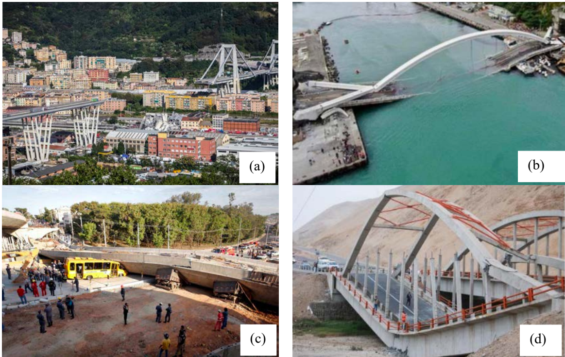
Figure 1.4. Structural bridge collapses around the world (a) Morandi Highway Bridge, Italy [26] (b) Nanfang`ao Bridge, Taiwan [28] (c) Guararapes Battle Viaduct, Brazil [29] (d) Topará Bridge, Peru [30].
